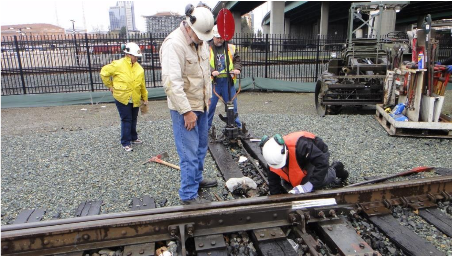
Now adjusted, Josh bolts the switch back together
