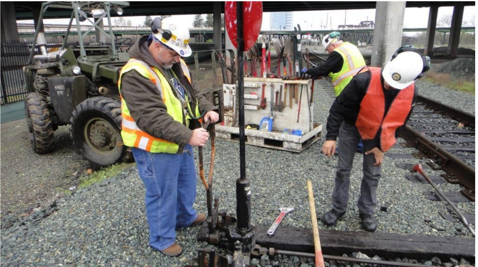
Mike F. centers the handle in order to set the new alignment
